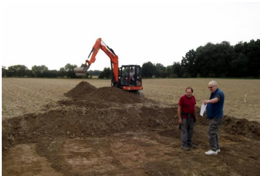
Figure 3 – Machine excavation in progress
